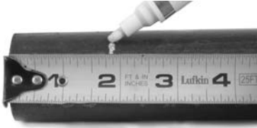
Figure 5A – Marking the Pipe Before Inserting Into Fitting Using Tape Measure
