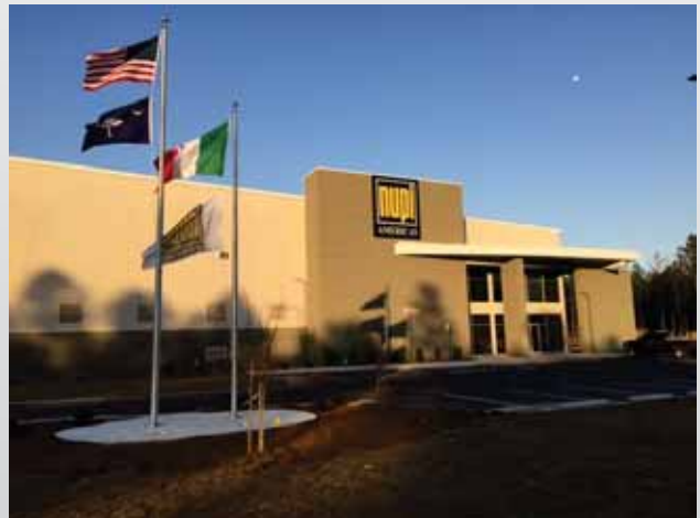
Nupi - Distribution & Fabrication Facility Early Branch, SC
